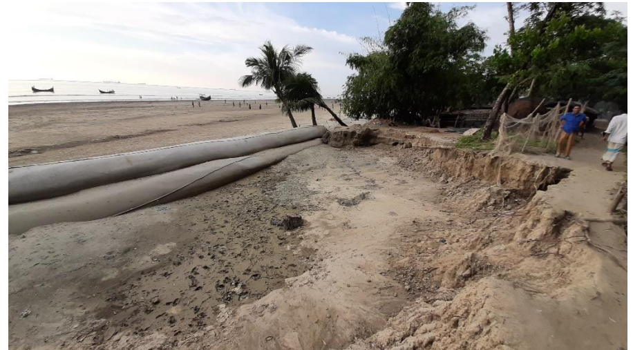
Figure 29: Broken part of the embankment in ward 8
