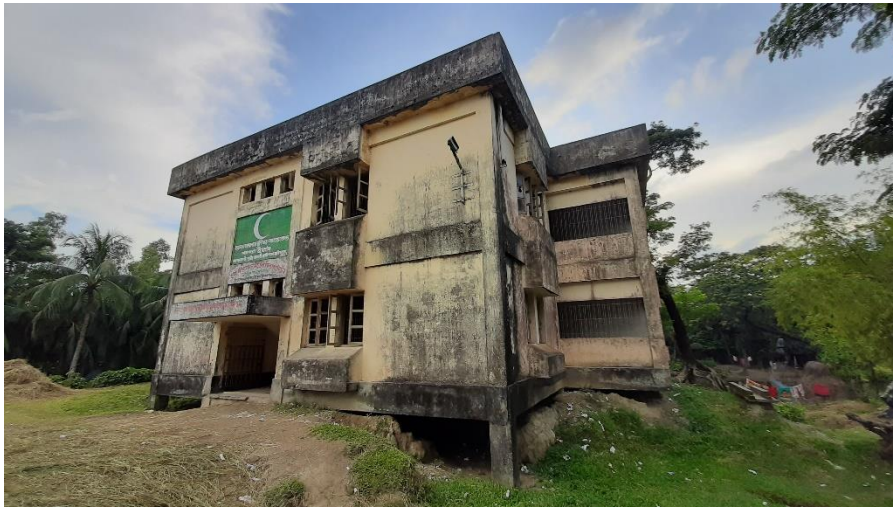
Figure 26: Cyclone Shelter in Killa that has no soil support in the base of the shelter
