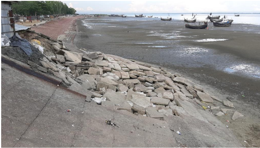
Figure 22: Broken part of the embankment in Ali Akbar Dail launch ghat
