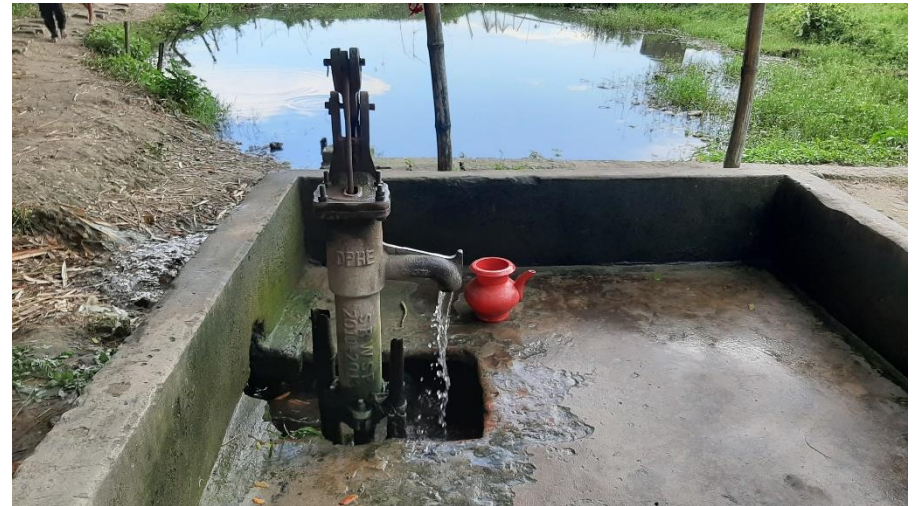
Figure 19: Deep tubewell where water is flowing nonstop
