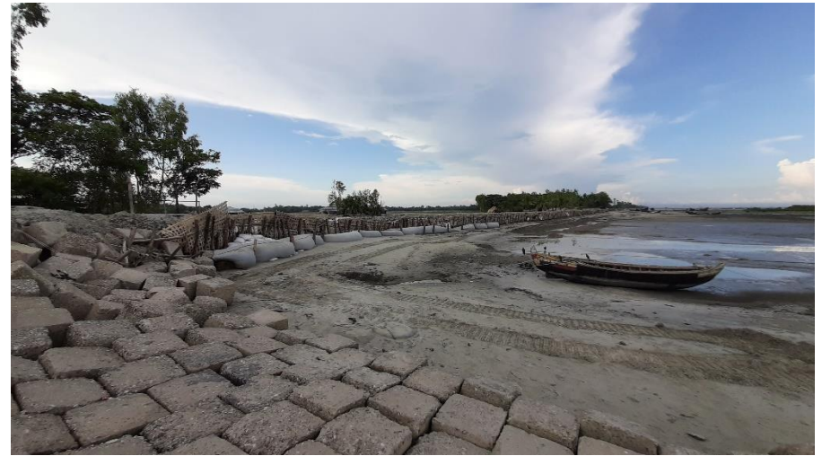
Figure 23: Broken part of the embankment beside Jelepara
