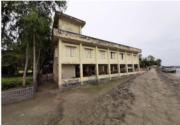
Figure 18: Primary school cum cyclone shelter beside the embankment
