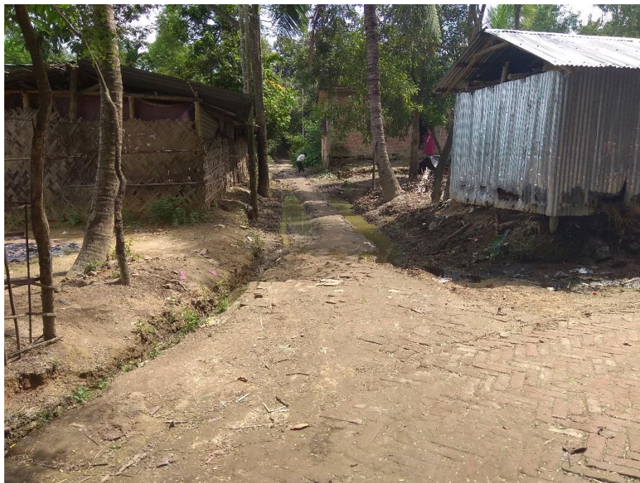
Figure 4: Hajirghona HBB (Herring Bone Bond) road (prone to flooding)
