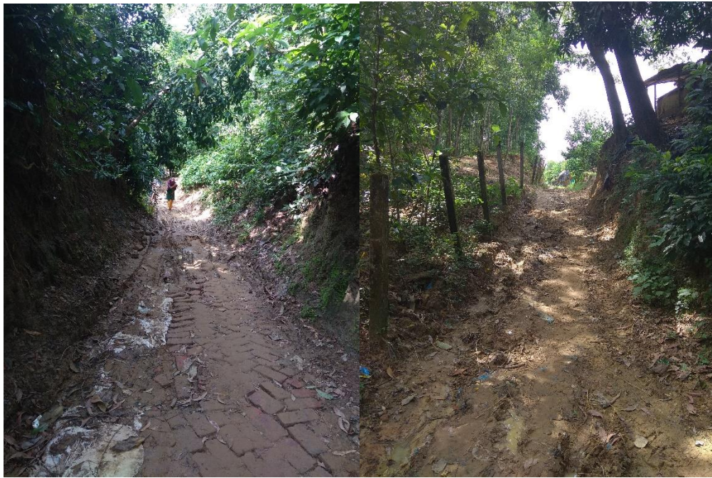
Figure 7: Tarabunia Para side road, in ward no 9 (prone to floods and flash floods)
