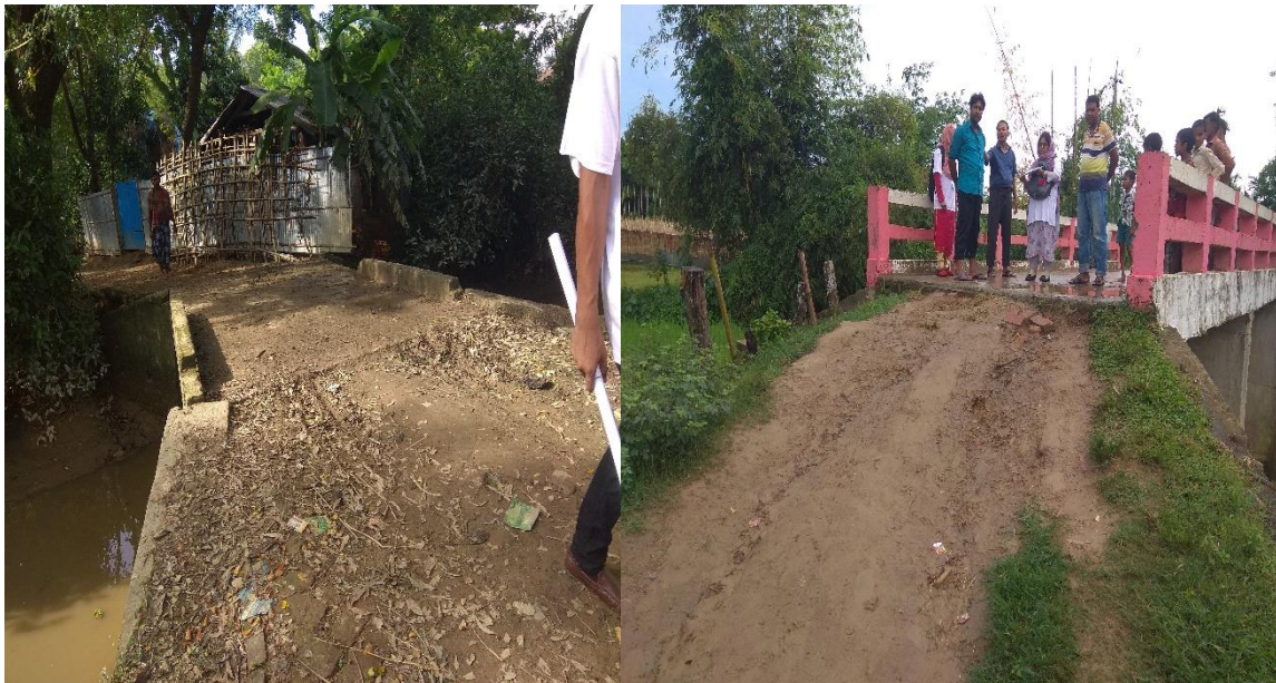
Figure 10: Shilkhali to Pekua connecting Shakoo in ward no 2 by southern side of Shilkhali High School (left), Dalar Mukher Culvert in ward no 6 (right)
