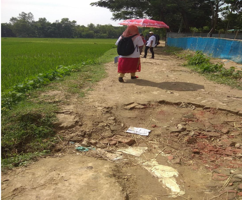
Figure 5: Petan Matbor Para Govt. Primary school road, 1.5 km flat soling and HBB (Herring Bone Bond) in ward no 9 (prone to flooding)
