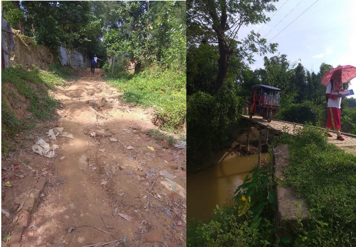
Figure 9: Dokan Para to Shobuj Para 1km HBB (Herring Bone Bond) road in ward no 7 (left); the shako situated in the western side of Hedayetabadi in ward no 2 (right)
