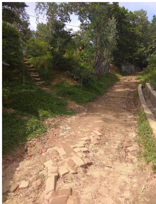
Figure 8: Shobuj para School Road, 400 feet, in ward no 7, HBB (Herring Bone Bond) road (prone to flooding)
