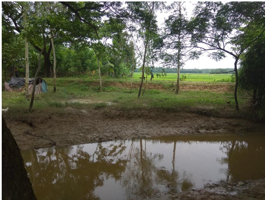
Figure 1: Highly sedimented Jarul bunia canal situated between wards no 4 and 7
