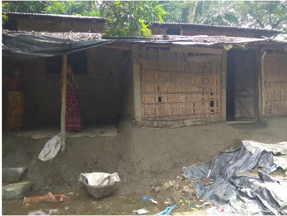
Figure 3: Hajirghona para of ward no 8 cluster village (prone to flooding around 4/5 feet water height)
