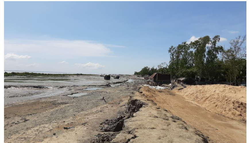
Figure 24: Broken part of the embankment in ward 6
