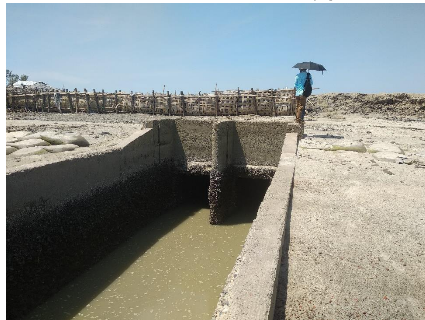
Figure 18: Broken sluice gate in ward 6
